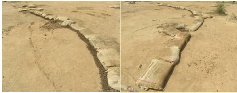
Figure 2: Bund structures with V-shaped microcatchment in the Maroua-Salak site at the beginning of the implementation in 2012
