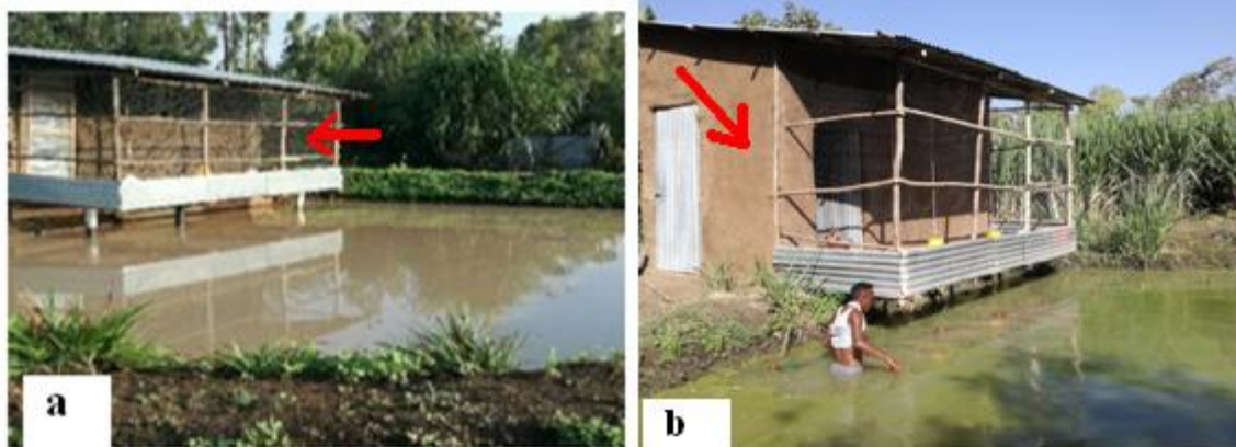
Figure 2: Constructed poultry house used for feeding and drinking during day time (a) used as a place to lay egg (b)
