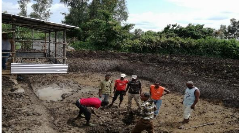
Figure 3: Fish pond construction under poultry house
