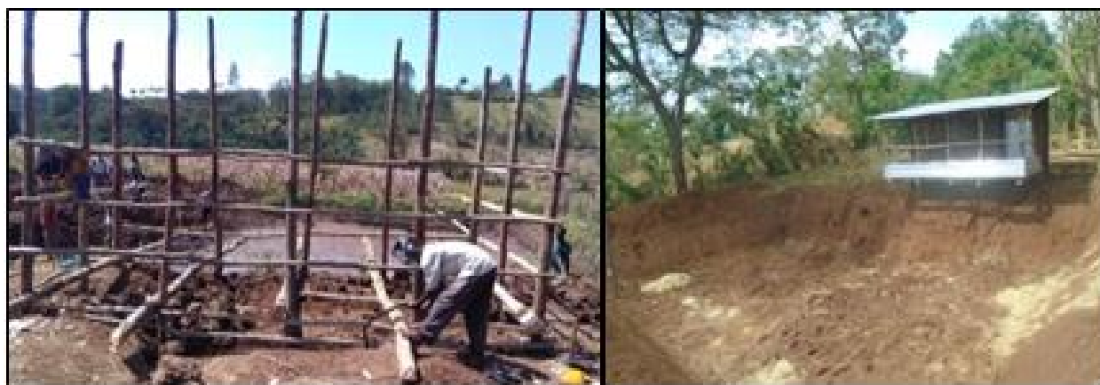
Figure 3. Poultry house construction hovering on fish pond
