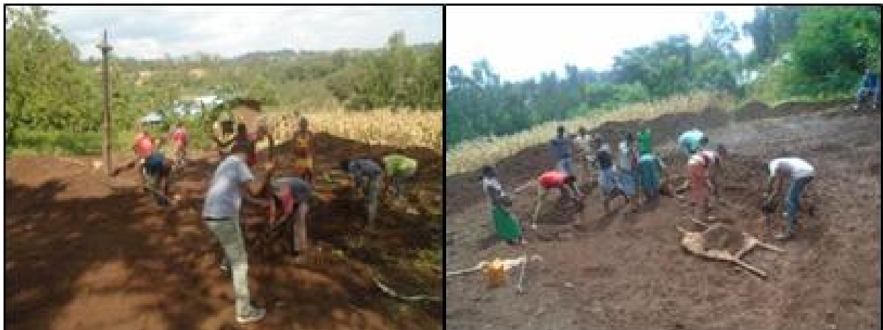
Figure 2. Fish pond construction under poultry house
