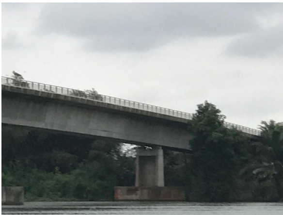
View of the bridge on left bank of the Kouilou River
